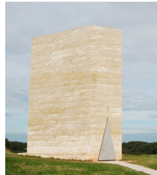
Fig. 7.33: use of rammed concrete at the Bruder Klaus Kapelle by Peter Zumthor in Wachendorf, Germany; source: Willem-Jan Beeren, 2011
