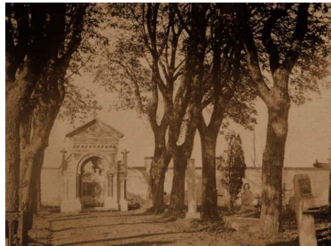
Fig. 6.15: The lane planted perpendicular to the main entrance gate. Source: gemeentearchief Maastricht via Denessen & Bruijnesteijn, 2002
