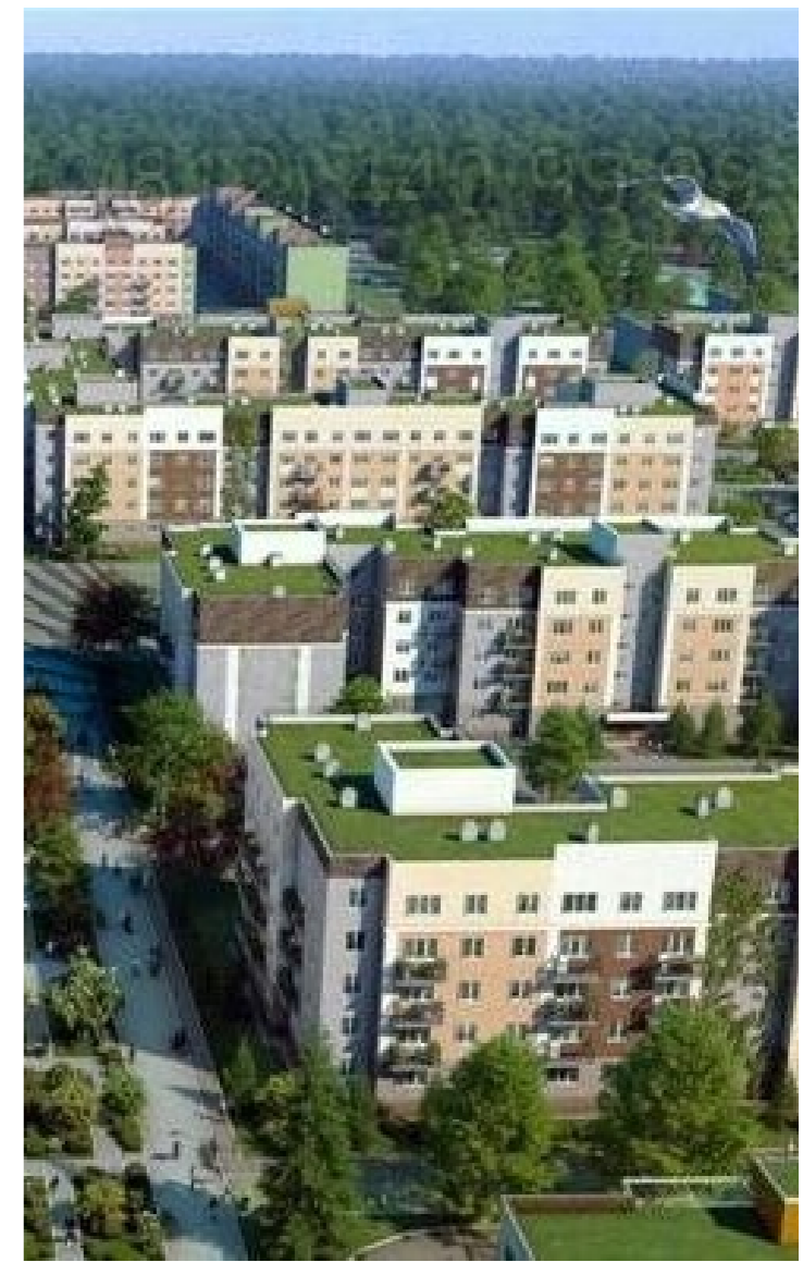
In the present day the city continues to expand, creating a stronger border with the nature by chipping more and more away from it.
